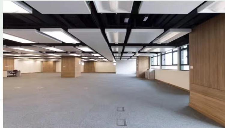
Radiant Cooling Panel and Dimmable Indirect LED Lighting
